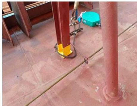
Figure 9 – Demonstration of an anchor point on deck with fall arrestor (Source: the Company)
